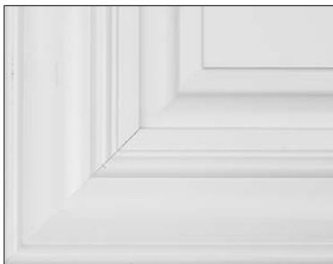
Example of front joint separation
