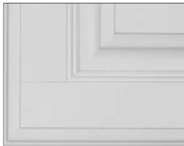
Example of front joint separation
