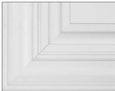
Example of front joint separation
