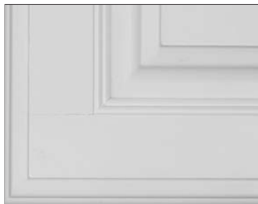
Example of front joint separation
