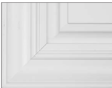
Example of front joint separation
