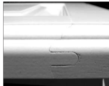
Example of end joint separation
