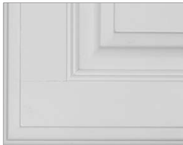
Example of front joint separation
