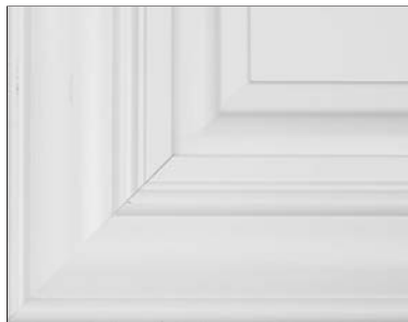
Example of front joint separation
