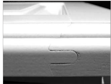
Example of door end joint separation
