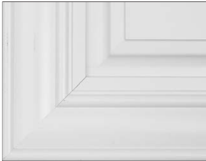
Example of door front joint separation
