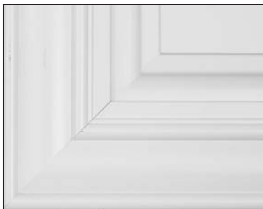
Example of front joint separation
